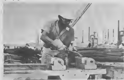
At the RE-BAR bending machine a Parsons employee wears goggles, heavy canvas gloves and apron for protection. Na mashin di dobla heru un empleado di Parsons ta usa bril di seguridad, handschoen diki y lantera pa su proteccion.
